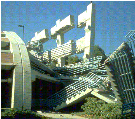
Cal State University Northridge Parking Structure after 1994 earthquake.
