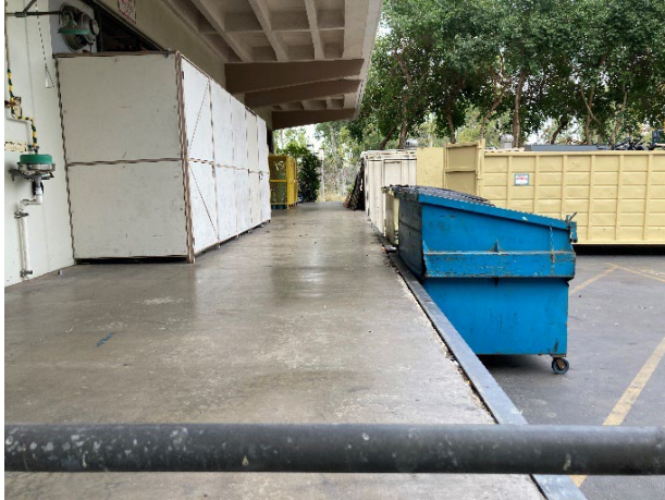
Trash Dumpster Without Railing
