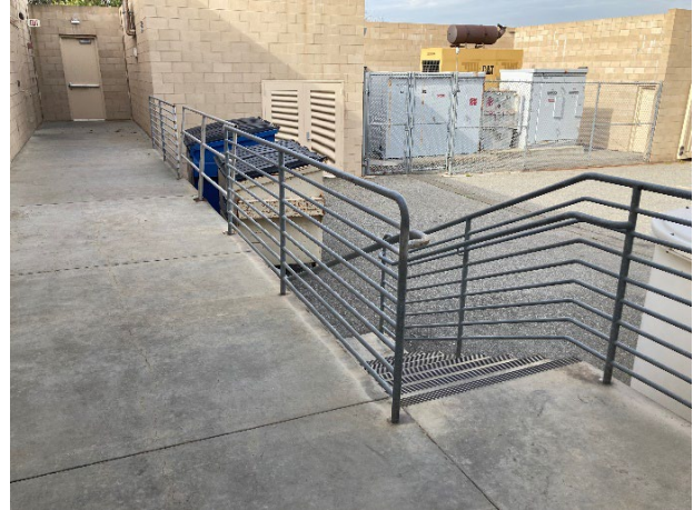
Trash Dumpster With Railing
